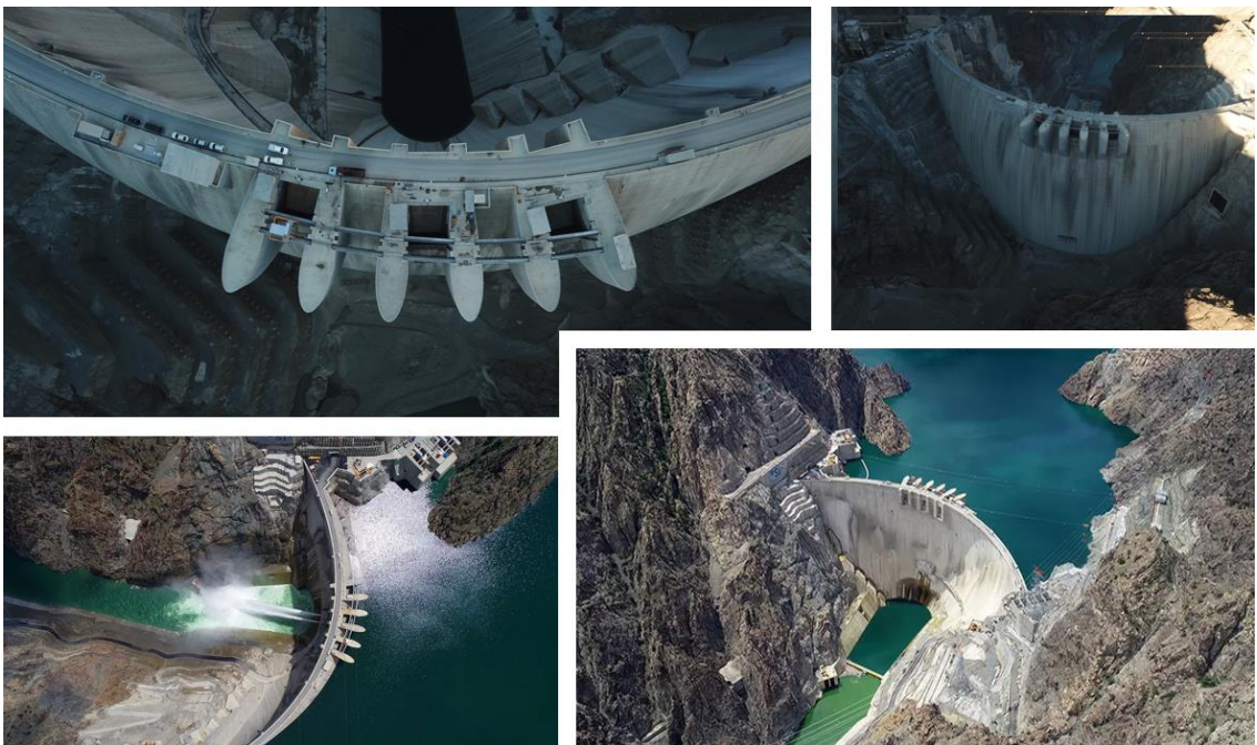
Fig. 1. The views of Yusufeli Arch Dam [19]
