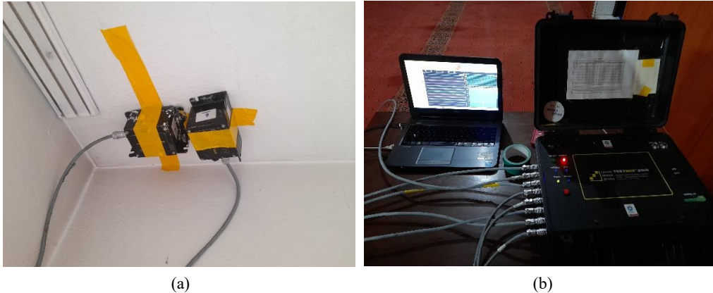
Fig. 9. Images from the response vibration measurement work within the scope of OMA applications: (a) accelerometer sensors; (b) data acquisition system
