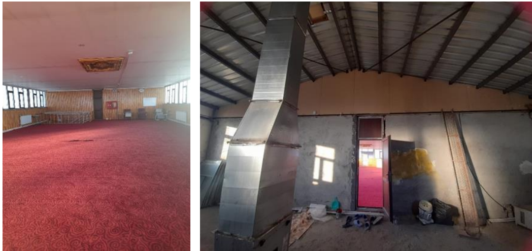
Fig. 3. Attic: Meeting area (Left), Partition wall and roof support system (Right)
