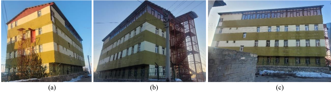
Fig. 1. Various views of the examined educational building: (a) southeast facade; (b) northeast facade; (c) east façade
