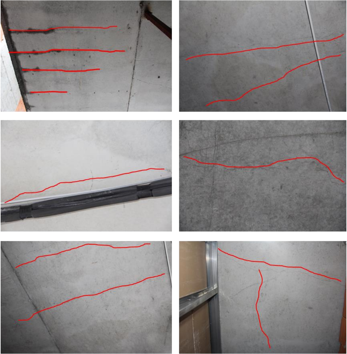
Fig. 1. Slab damages
