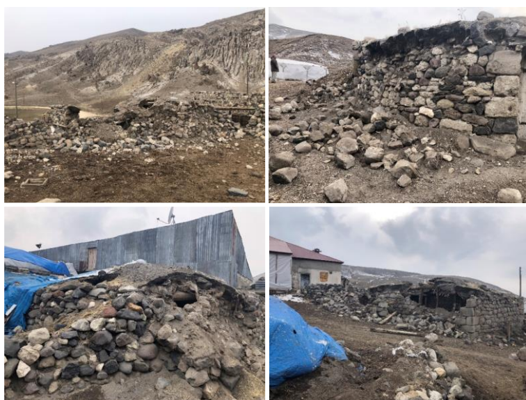
Fig. 12. Collapsed masonry structures
