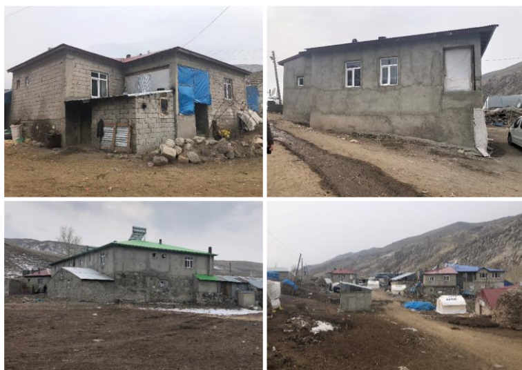
Fig. 13. Undamaged reinforced concrete structures
