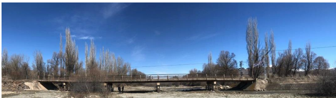
Fig. 5. Picture of bridge
