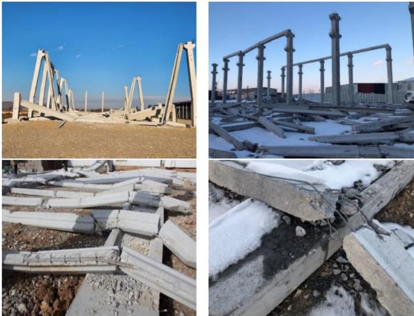
Fig. 20. The damages on steel industrial structures
