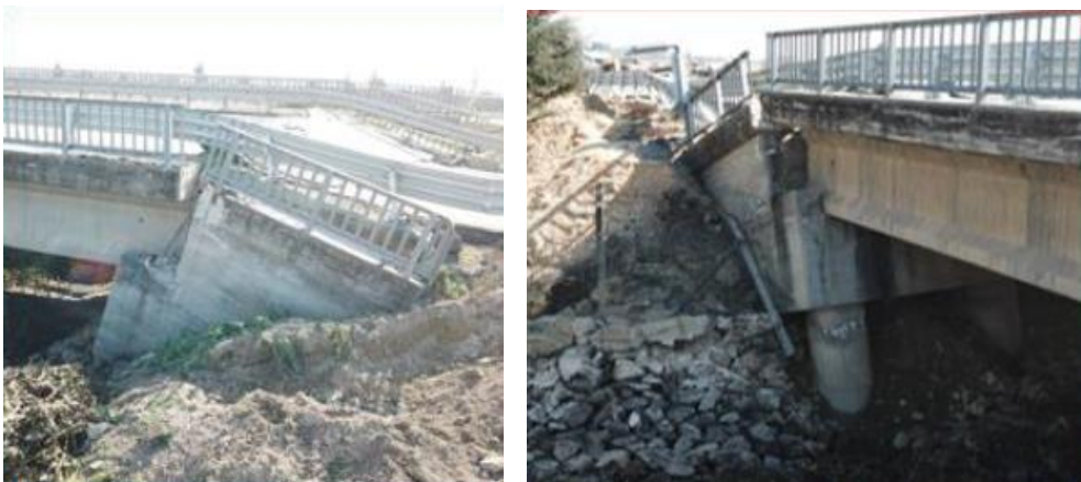
Fig. 21. Ground-foundation damages
