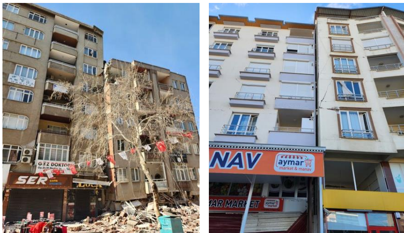
Fig. 10. Inadequate safe distance
