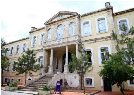
Fig. 2. Monumental Entrance Facade
