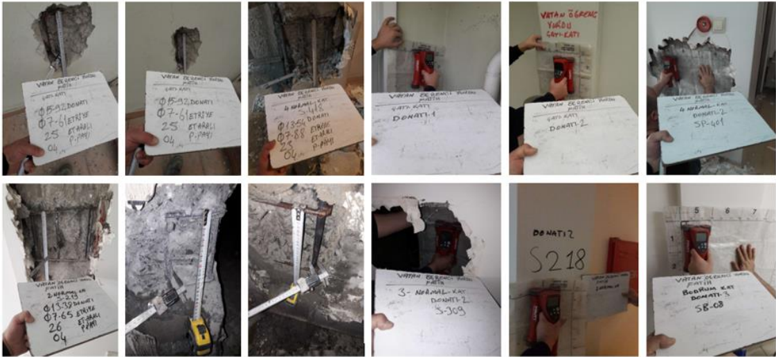
Fig. 5. Rebar examination using destructive and non-destructive techniques
