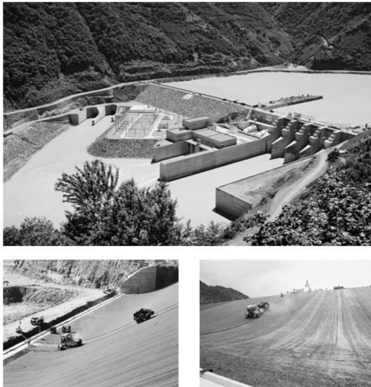
Fig. 2. Muratlı Dam constructed in Artvin, Turkey
