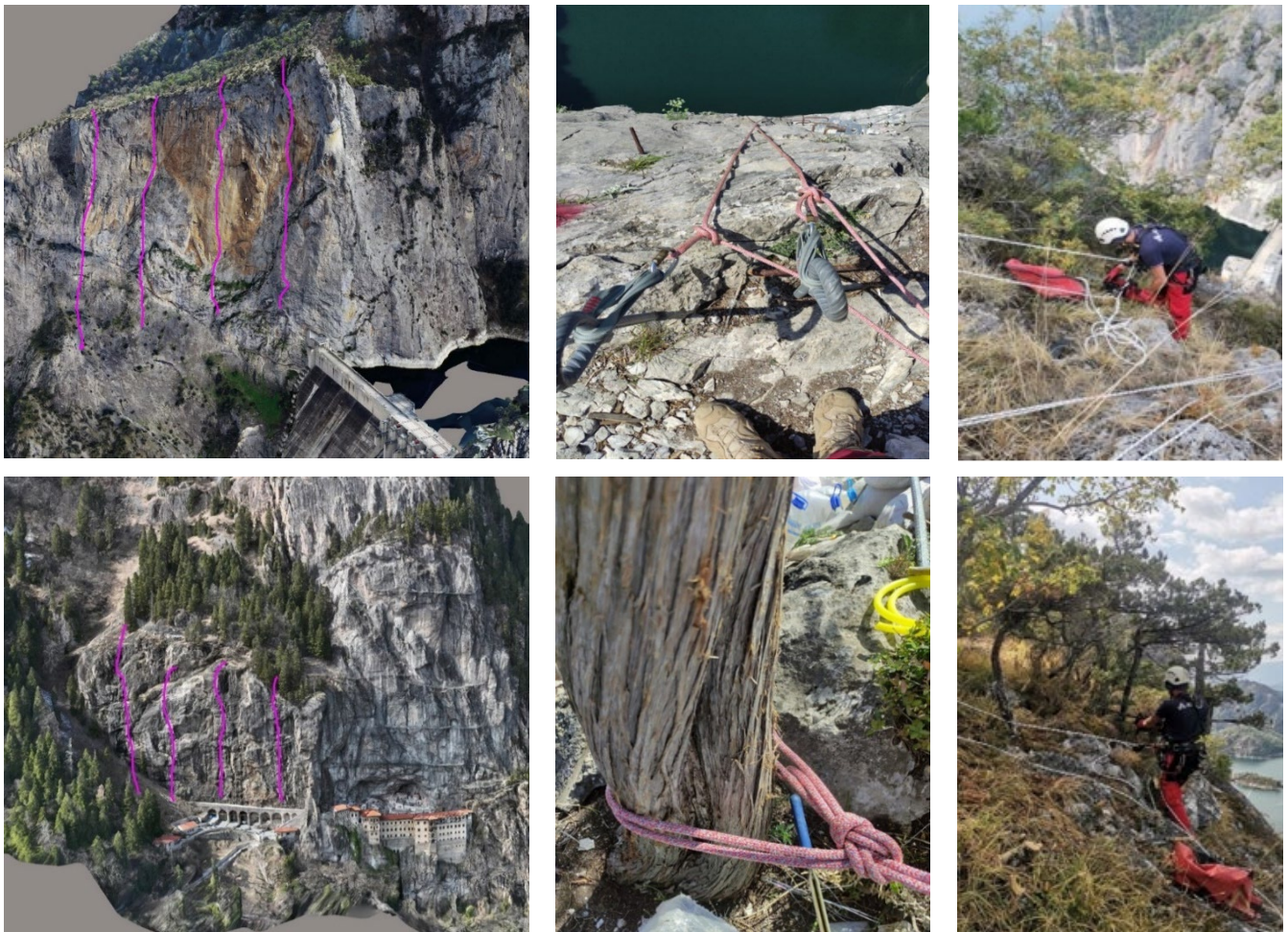
Fig. 12. Rope-access routes, anchorage zones, and surface cleaning stages in rockfall mitigation projects
