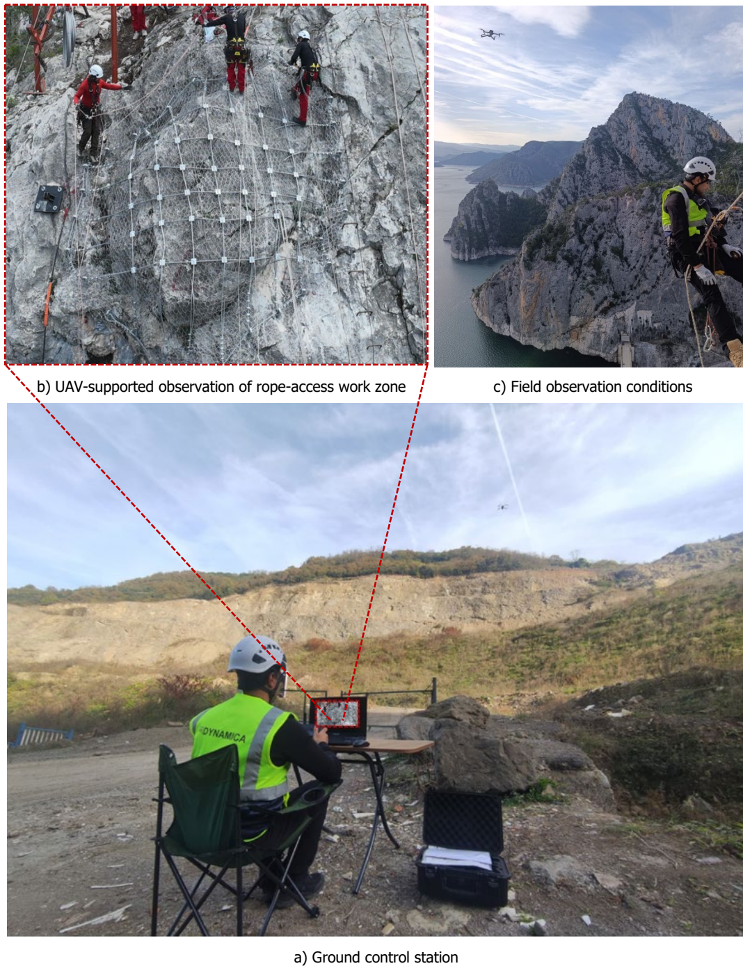
Fig. 14. Pilot implementation setup showing the ground control station and UAV-supported field observation conditions
