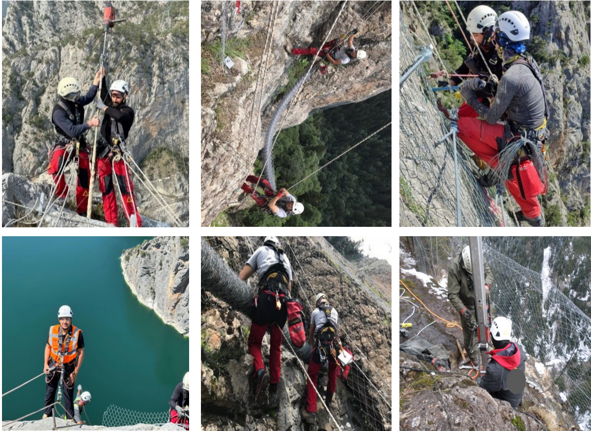
Fig. 1. Field conditions and rope-access operations observed in active rockfall mitigation projects
