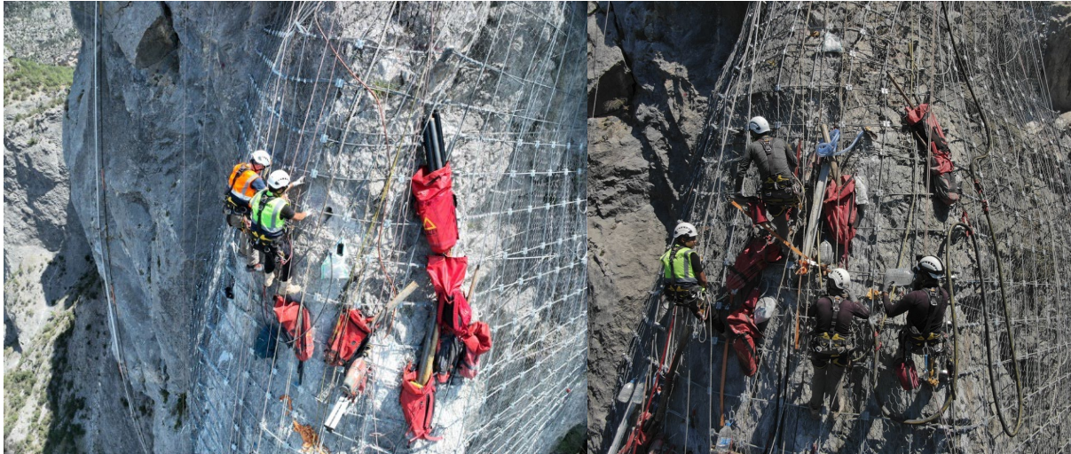
Fig. 13. Examples of UAV-supported visual observation of rope-access activities and equipment-related field conditions
