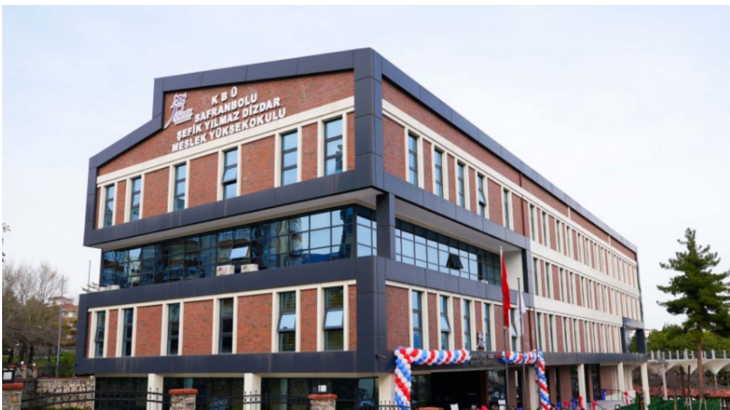
Fig. 1. Building of Safranbolu Şefik Dizdar (S.Ş.D.) Vocational School of Higher Education
