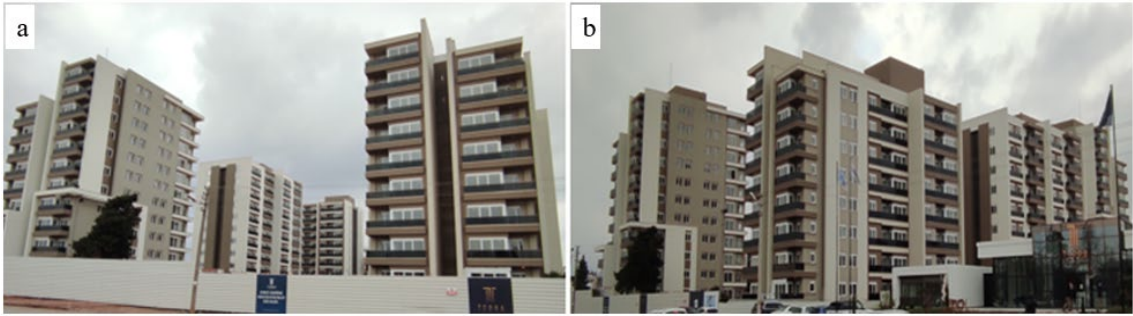
Fig. 7. Photograph of the island-based settlement project study area (a) Block F south facade, (b) Block F south facade east facade
