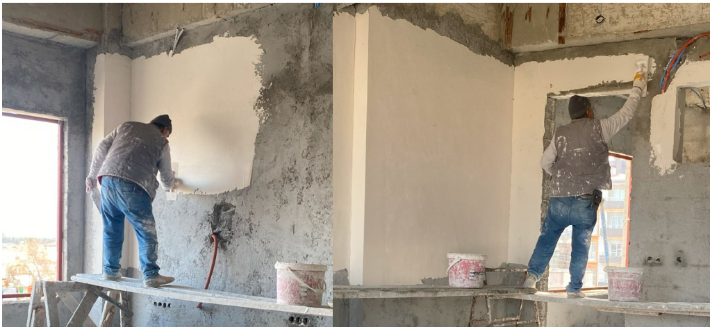
Fig. 3. Data collection with a sensor attached to the gypsum plaster workers' arm
