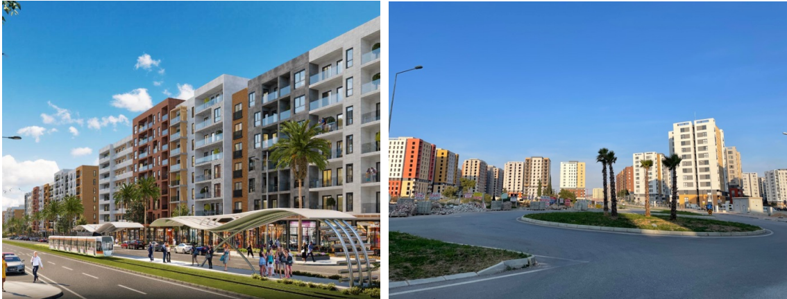
Fig. 6. Left: The tram line is planned to pass through the area in the project [19]; Right: Buildings and roads under construction
