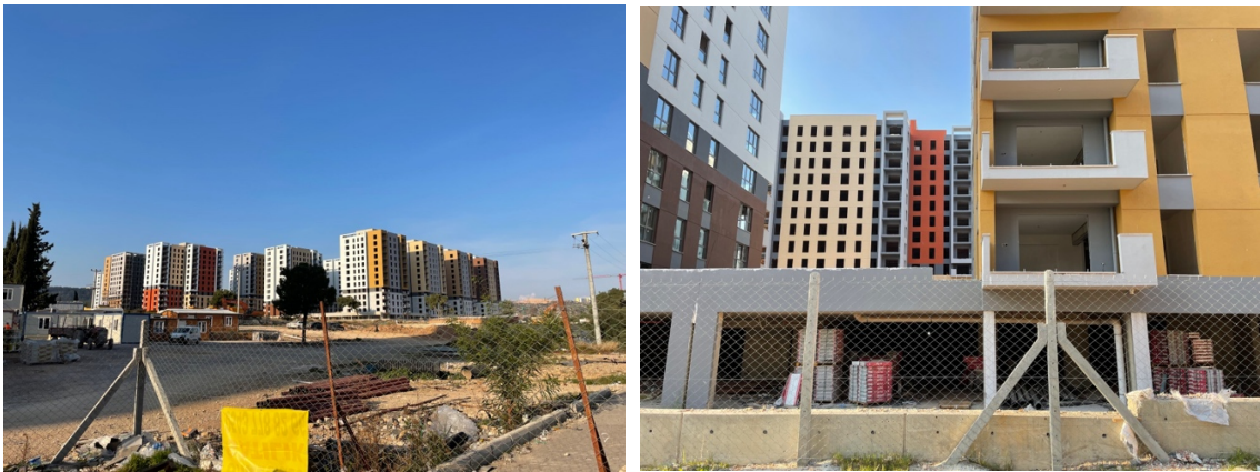
Fig. 7. Left: Buildings under construction and their environment; Right: Buildings under construction
