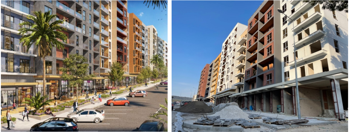
Fig. 5. Left: Commercial areas and residences in the project [19]; Right: Commercial areas and residences under construction
