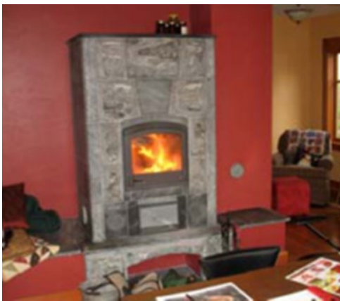
Fig. 2. Contraflow masonry heater [12]
