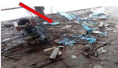
Fig. 4. Lack of waste management system
