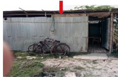
Fig. 5. Unplanned location of site office
